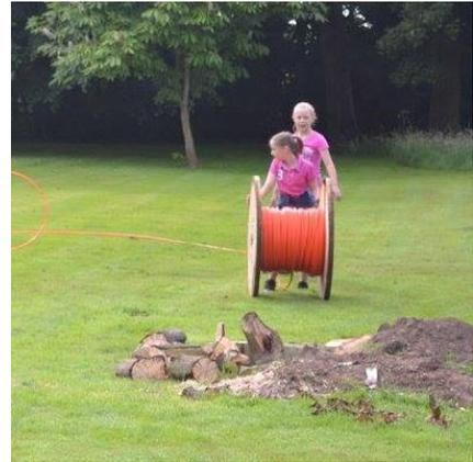
4. Close to the property we need to change from the orange duct (which has to be buried) to a black duct that can be run above ground. We will install the joint for you - so it needs to be left exposed when the rest of the duct is buried.
