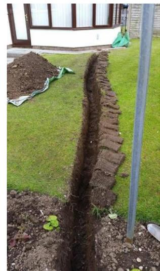
3. We will provide the ducting - lay this in the trench making sure that it's reasonably straight and is not going to be damaged by sharp stones. Consider sieving the soil back over the duct or laying it in some sand.
