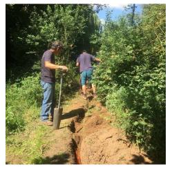
spade, but remember that the duct will be there for many years so make sure you know where it is and it's not somewhere that you expect to be digging again any time soon! The trench needs to be reasonably straight as we have to blow the fibre through the duct does not like going round bends.
