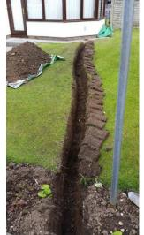
3. We will provide the ducting - lay this in the trench making sure that it's reasonably straight and is not going to be damaged by sharp stones. Consider sieving the soil back over the duct or laying it in some sand.
